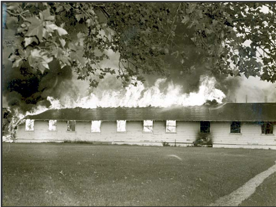
1967: Immolation of the old barracks style clinical research annex to make room for the long predicted new building
